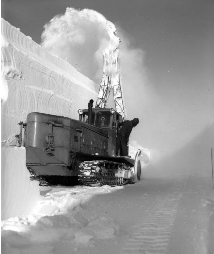
Figure 8.2 The Peter Snow Miller in operation cutting a trench in the ice. US Army Photos (public domain).
