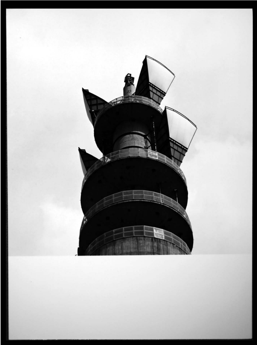
Figure VE 3.15 Close-up view of the horn reflectors on the Heaton Park microwave tower, 1966.
