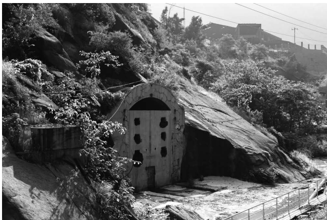
Figure VE 1.4 A sealed hillside entrance to the decommissioned Power Plant 503 in the Panzhihua area. The plant started to operate in the mid-1970s, and was considered as the state of the art at the time with all its facilities concealed in a vast tunnel system.
