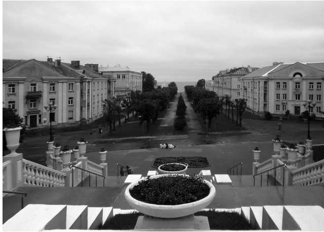
Figure 3.6 Stalinist centre of Sillamäe, view from staircase along Mere Boulevard, early 1950s, by Lengorstroyproyekt / GSPI-12 . Photograph taken in 2013. Source: Siim Sultson.
