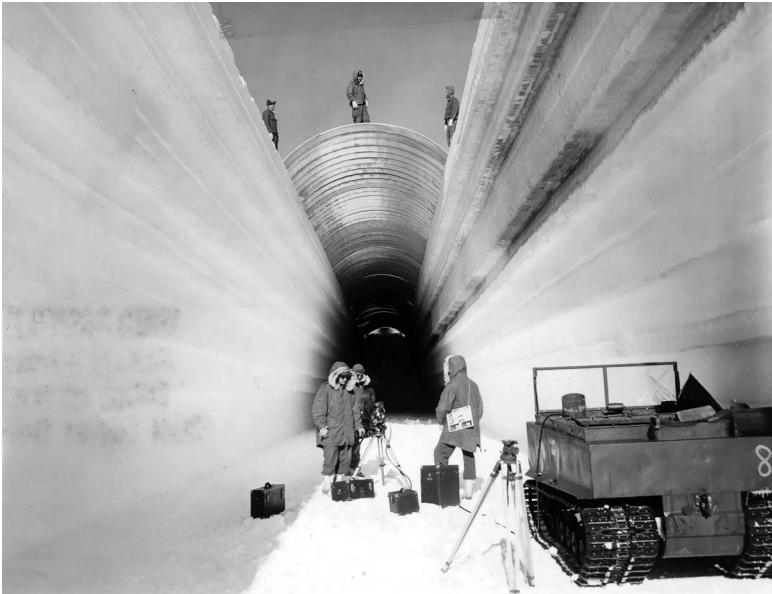
Figure 8.3 Trench partially covered with steel arch roofs. The US Army Signal Corps' Pictorial Service team is filming in the trench. US Army Photo (public domain).
