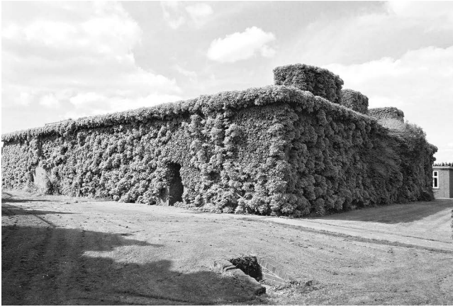
Figure 2.3 The War Room at Flowers Hill, Bristol. This protected structure was the seat of Home Defence Region 7s Regional Commissioner on transition to war.
