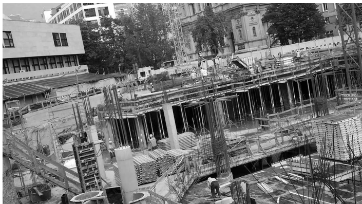
Figure 5.12 Construction of metro line II using cut-and-cover technique, 2014. Source: Author's photograph.
