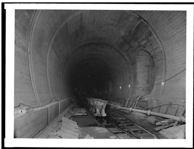
Figure VE 3.2 Part of the main tunnel fully lined with concrete, connection to side tunnel evident, 1956.
