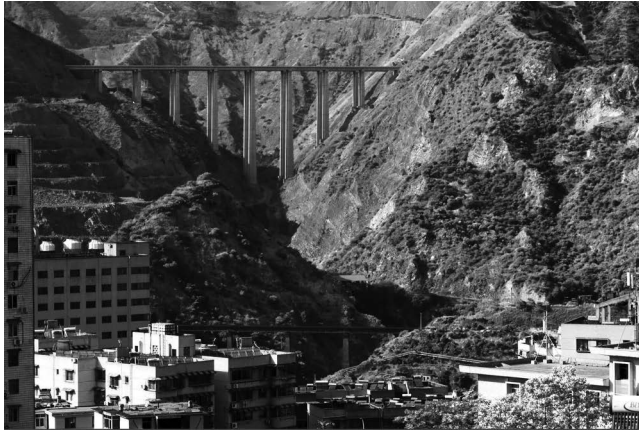
Figure VE 1.2 Traversing the mountains high above the city of Panzhihua is one of the many rail bridges from the Chengdu-Kunming Railway, which linked major Cold War cities in south-western China. Completed in 1970, the 1134 km railway was regarded as a major Third Front achievement.
