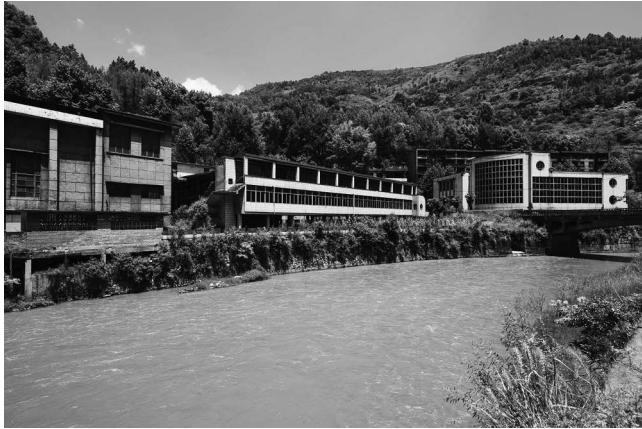
Figure VE 1.3 Factory 300 was one of the several major power plants that supported the heavy industries in the Liupanshui area. Its canteen, market, hospital, school, park, workers' dormitories, as well as power generating facilities were built along a river, making it a typical ribbon-shaped Third Front factory town.
