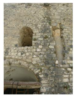
**Figures 11.6b–c** The war inflicted great structural damages to the mosque, revealing older pillars from a previous structure buried within its walls. These remnants might be seen as indicative of a unique preservation approach that opted not to tear down, but rather to build on. Image: Marwa al-Sabouni
