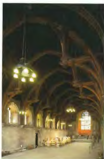
London, Westminster Hall, Houses of Parliament Hammerbeam roof (1394–1401) by master carpenter Hugo Herland
