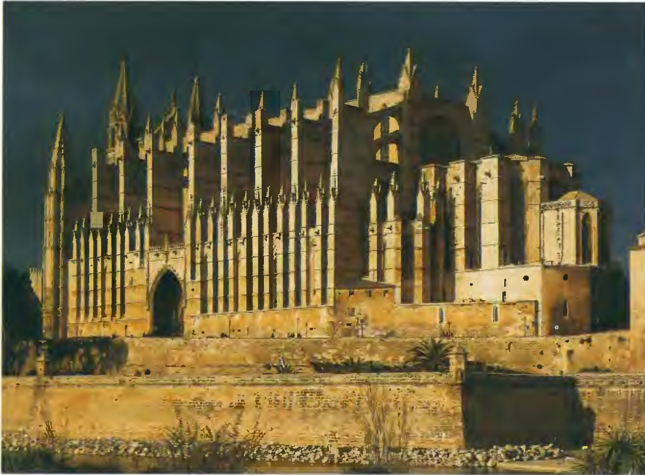
TOP LEFT AND OPPOSITE: Berenguer de Montagut (?) and others Palma de Mallorca, Cathedral of Santa Maria, begun ca. 1300 Exterior (left) Interior (opposite), 1369
