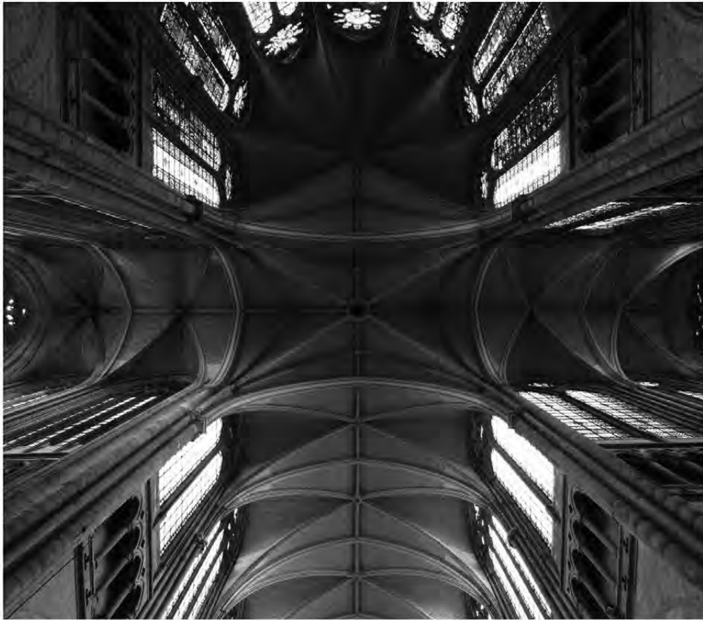
Fig. 4. Saint-Quentin, interior, vaults of eastern transept (Yves Gallet).
