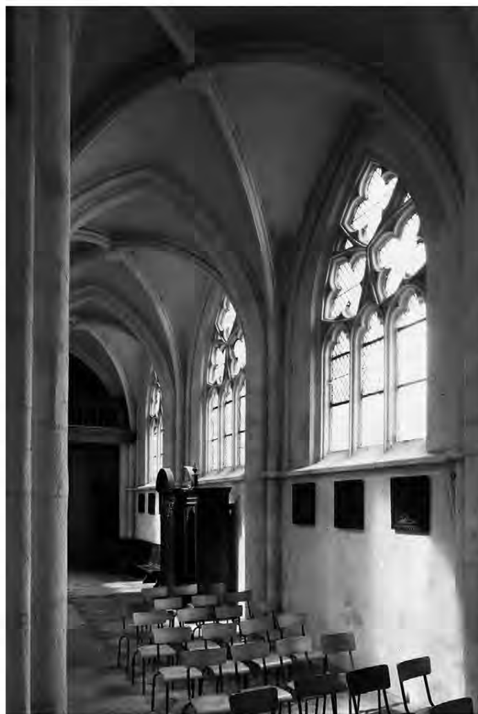
Fig. 2. Pont-à-Mousson, former church of the Order of St Antony, view from the east into the north aisle (Markus Hilbich).
