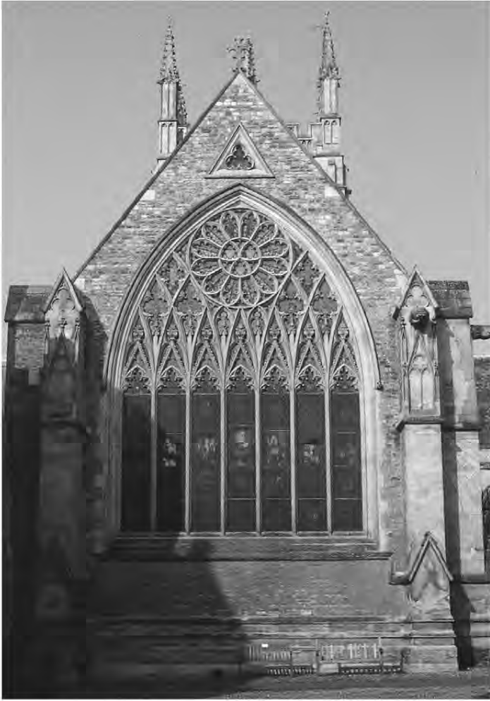
Fig. 2. Merton College Chapel, east window, exterior (Tim Ayers).
