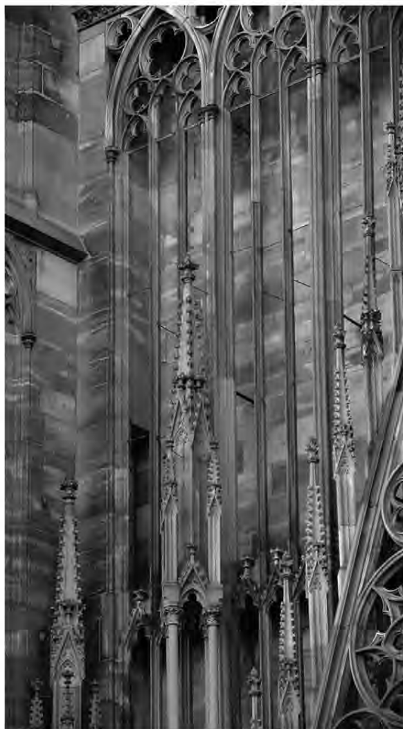
Fig. 4. Strasbourg Cathedral, tracery of the west façade, detail (Marc Carel Schurr).
