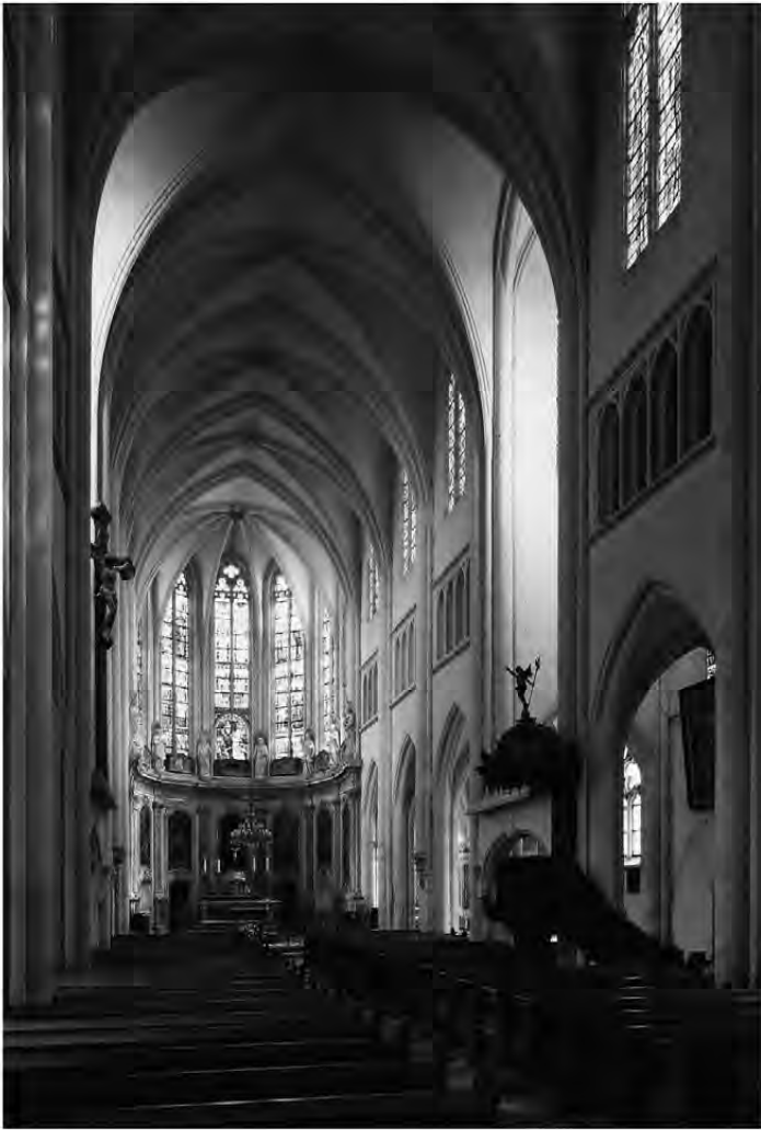
Fig. 1. Pont-à-Mousson, former church of the Order of St Antony, view to the east (Markus Hilbich).
