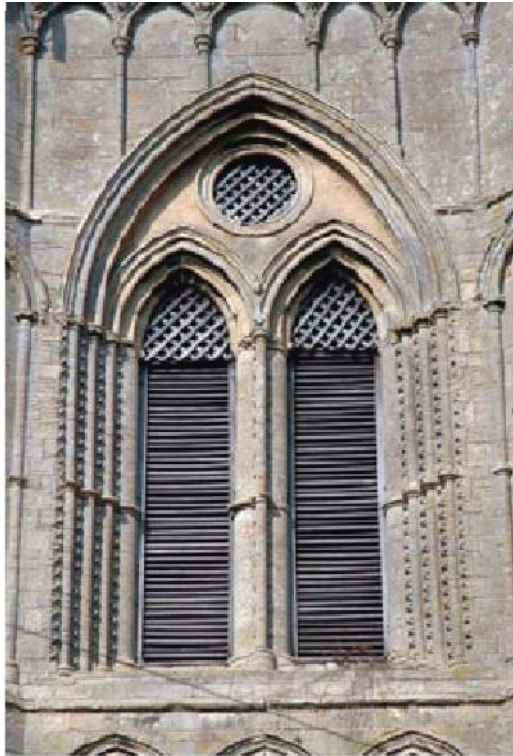
A typical plate tracery pattern: paired lancets, with a circlet above them, under a single arch.
