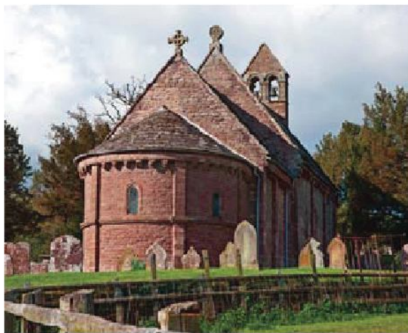
The church at Kilpeck, Herefordshire, is small, but perfectly proportioned. Its apse, shallow, flat buttresses and emphatic corbel table help mark it out as twelfth-century.
