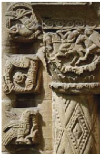
A lavishly sculpted Norman cushion capital on the doorway at Iffley, Oxfordshire. The chevron motif
