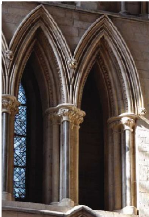
The attenuated form of the lancet arch: Lincoln Cathedral, early thirteenth century.
