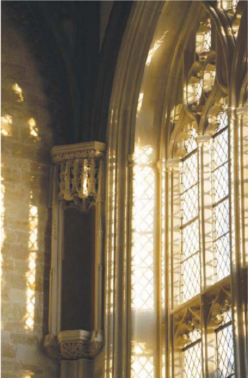
This niche, in the chapter house at Exeter Cathedral (after 1413) has a typically Perpendicular flat-topped profile.
