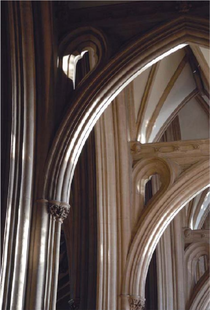
Small capitals clasp the diminutive shafts, while a great swoop of wave moulding runs continuously up the pier and into the arch. This pioneering design at Bristol Cathedral, possibly dated as early as 1298,
