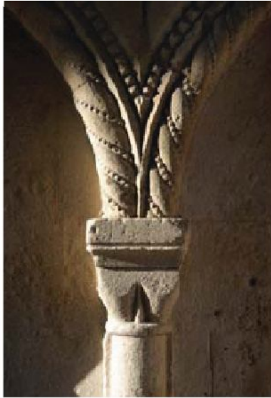
A capital divided into two or more cushions is a scallop capital; early nailhead can also be seen here, at the abbey gatehouse, Bristol Cathedral, c.1160.
