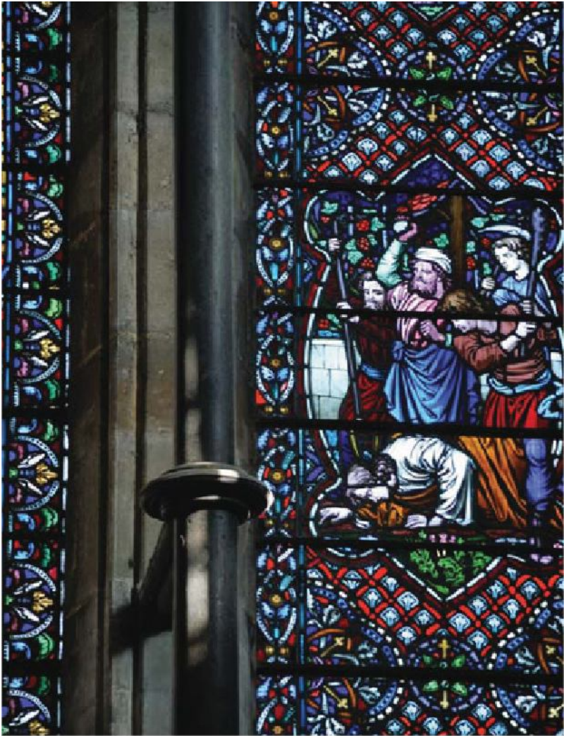
An en-delit shaft of polished Purbeck marble, clasped with a shaft-ring to mask joints in the stonework, at Boxgrove Priory.
