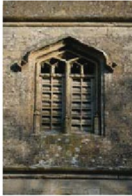
An emphatic drip-mould and a Tudor arch at Elkstone, Gloucestershire; fifteenth or sixteenth century.
