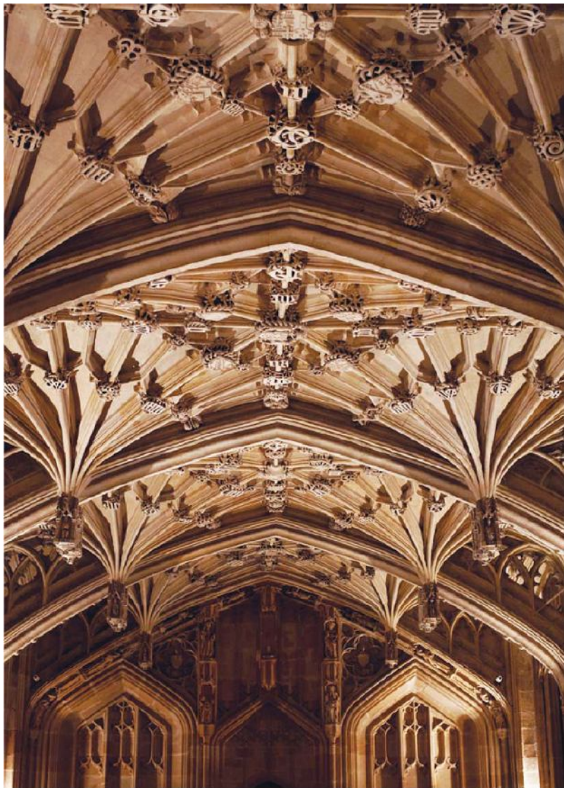
Tudor arches (in the three main blank arches) and pendant vaults at the Divinity School, Oxford (c.1423–83), a building that helped inspire a rebirth of architecture in the decades before the Reformation.
