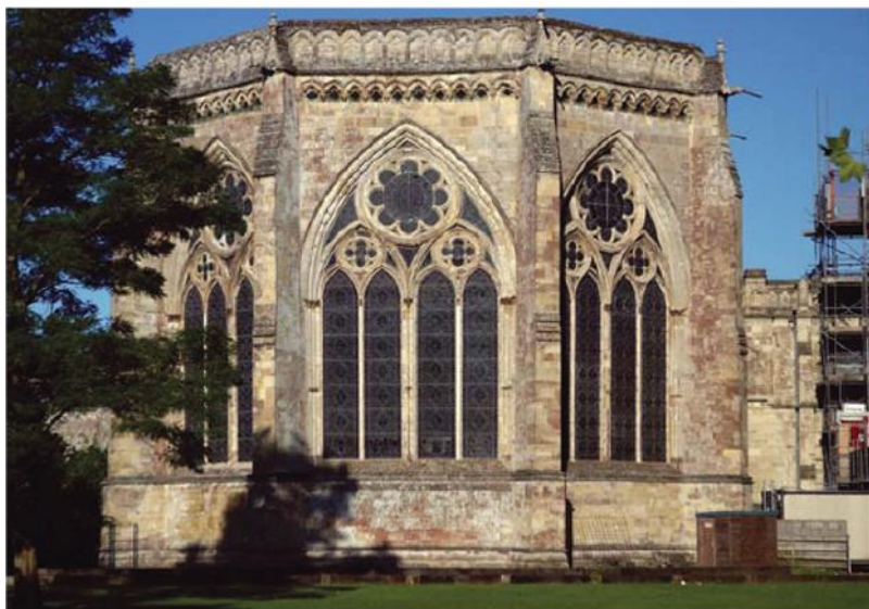
Four-light bar tracery, a tessellation of the two-light pattern, on the chapter house at Salisbury Cathedral (before 1263). The resulting pattern contains two sub-arches.
