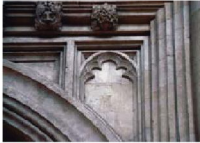
A panel in the nave at Winchester Cathedral (1370s–1394 to c. 1400), rising from the curved side of the arch beneath.
