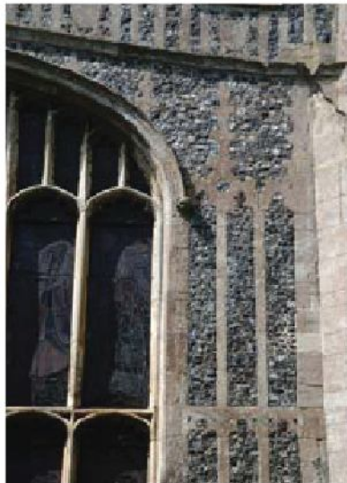
Panelling rendered in flushwork at Lavenham, Suffolk (1525).
