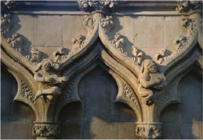
Ogee arches, lavishly sculpted, on the blank arcades at Beverley Minster, East Yorkshire (c. 1335–40).
