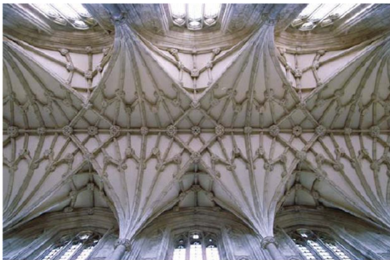
The vault in the nave at Winchester Cathedral (1370s–1394 to c. 1400) uses liernes to insert panel-like patterns between the tiercerons.
