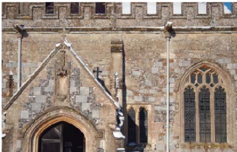
The three-light window on the right, at Avebury, Wiltshire, features what is probably the commonest Perpendicular tracery pattern of all: a pair of Perpendicular reticulations, each filled with two small
