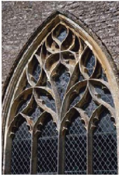
A Curvilinear window at Ducklington, Oxfordshire, probably c. 1320–40: ogee curves give a flowing quality to its tracery. Sub-arches divide the window into two halves. The areas of solid masonry in the uppermost motif carry sculpted statuary inside the building, a typically Decorated conceit.
