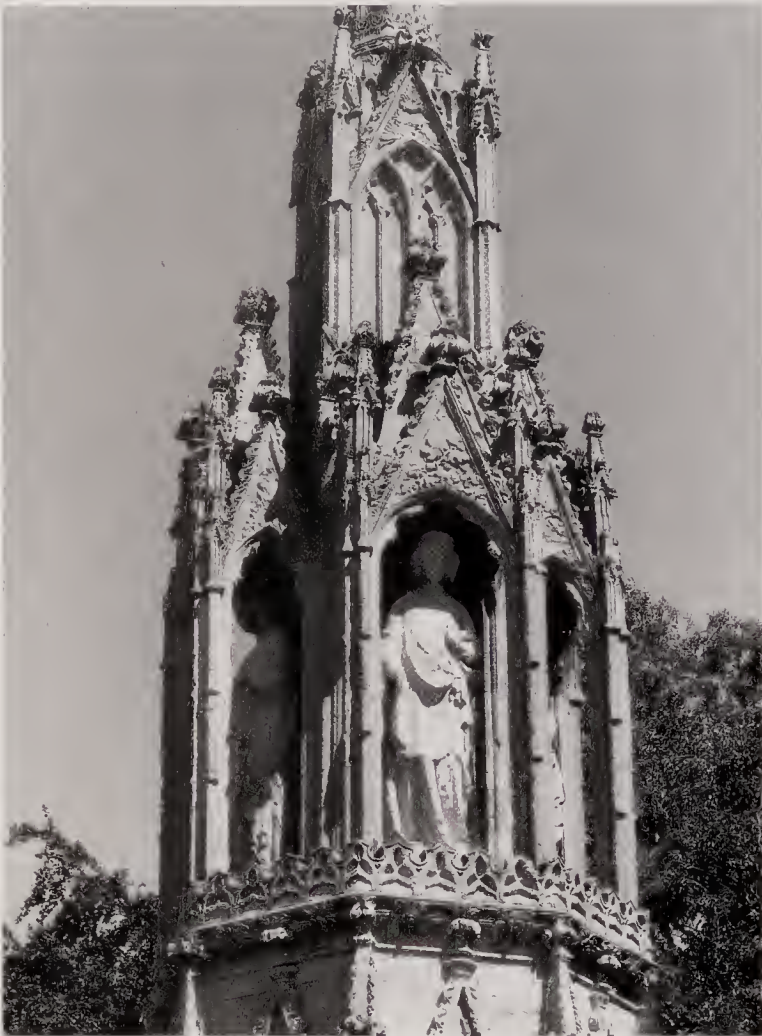
198. Hardington, Northamptonshire, Eleanor Cross, 1291–4
