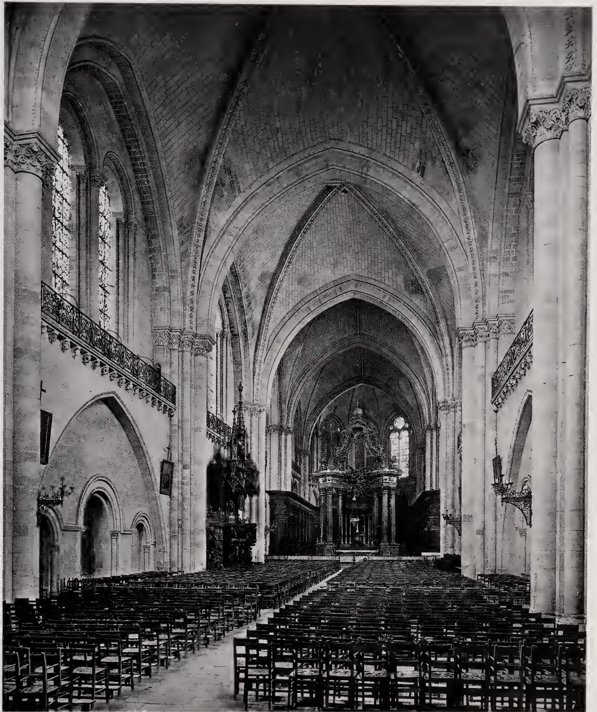
63. Angers, Saint-Maurice. Interior of nave, after 1149
