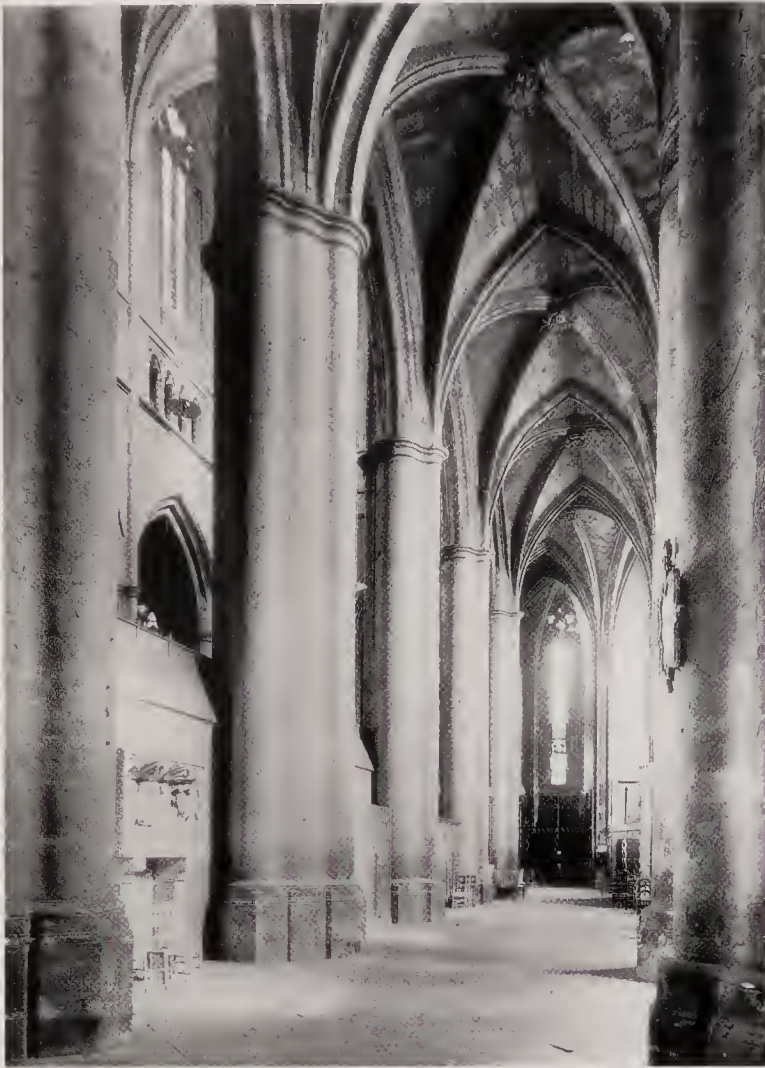
260. Rodez Cathedral. Choir aisle; three easternmost piers part of the chevet begun in 1277; pillars to their west, 1447; crossing piers 1462
