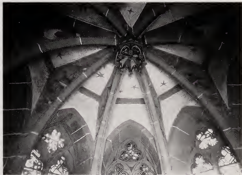
294. Calw, chapel of St Nicholas. Vaulting, c. 1360 (?)
