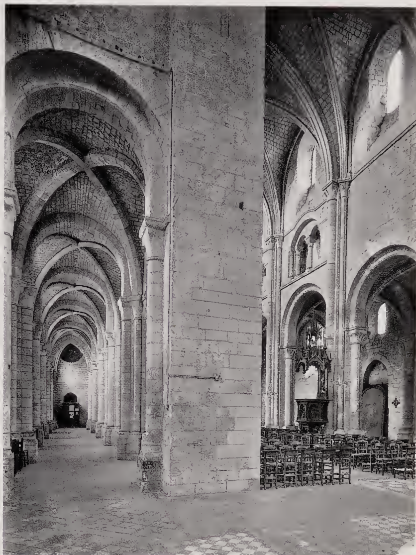
24. Beauvais, Saint-Etienne, begun c. 1120. Interior of the nave looking west. In the south aisle the nearest (earliest) vault has bevelled ribs, those further west have roll mouldings
