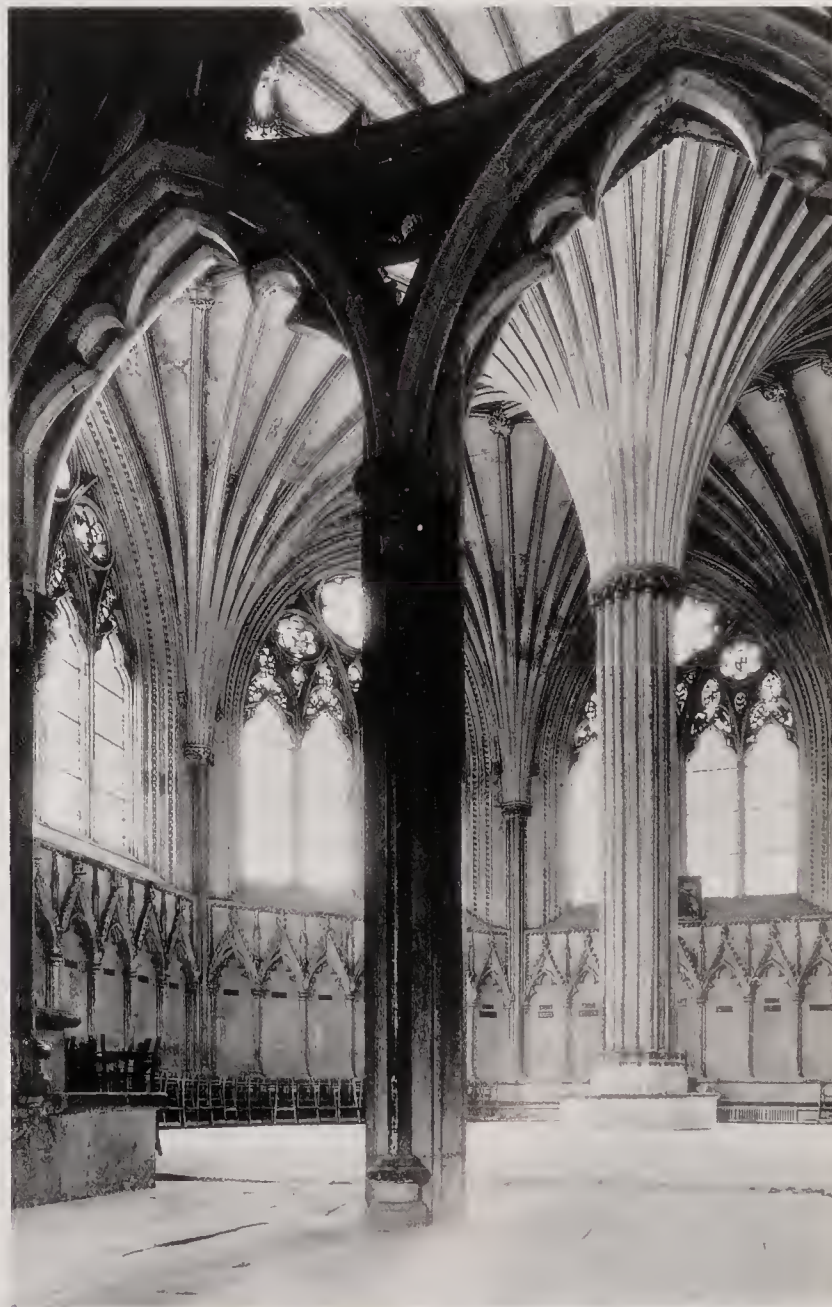
192. Wells Cathedral. Chapter House, upper chamber. Begun 1298, finished by 1305
