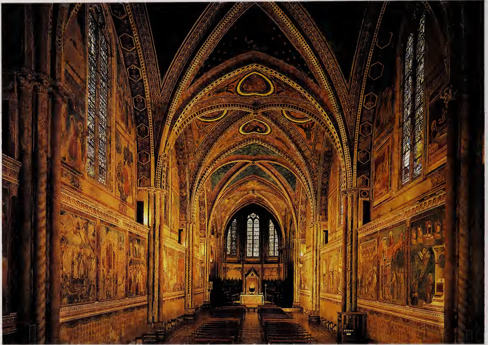
144. Assisi, S. Francesco, 1228–53. Interior of upper church, looking west
