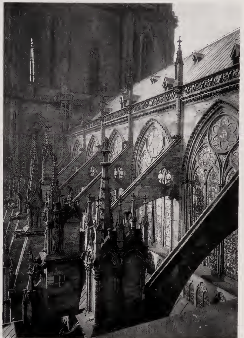
108. Strasbourg Cathedral. Flying buttresses of nave, begun after 1240
