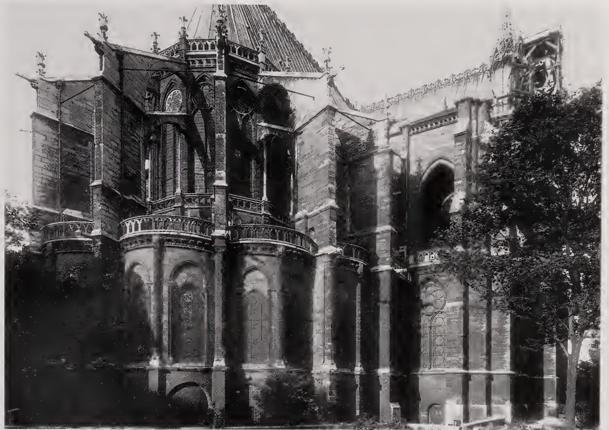
96. Saint-Denis Abbey Church. Exterior of choir, 1140–3 (radiating chapels) and 1231 onwards
