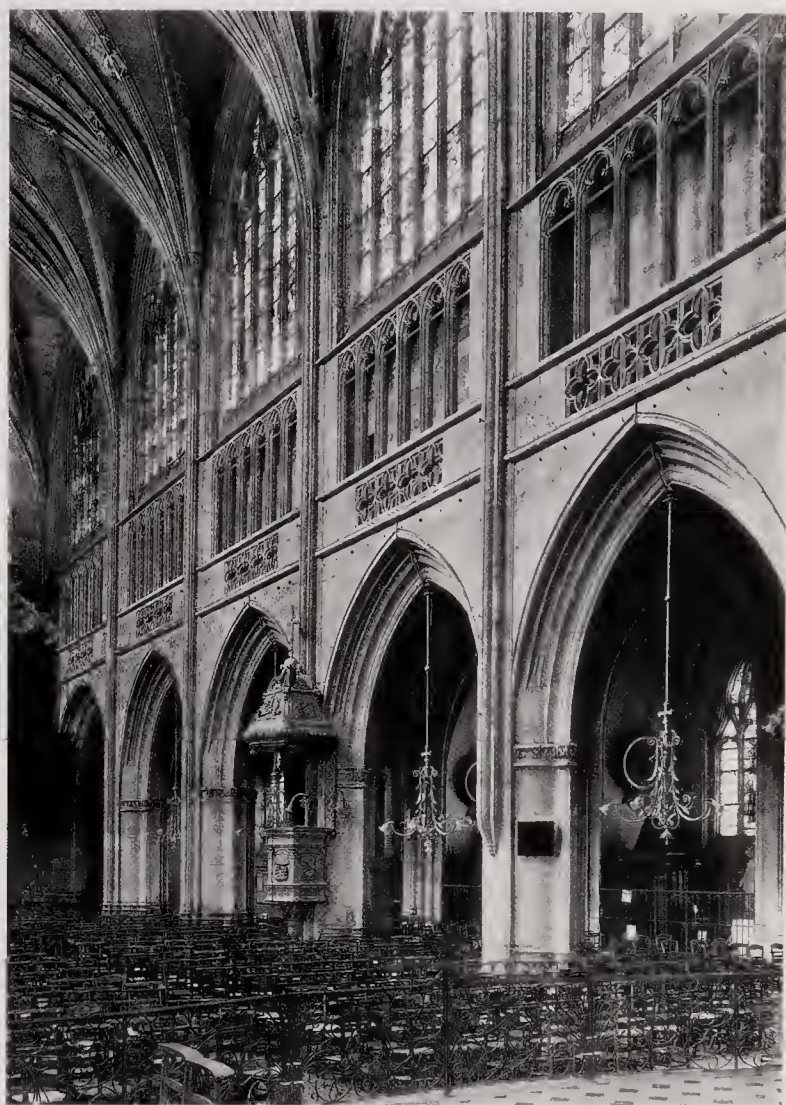
280. Alençon, Notre-Dame. Interior of nave, begun c. 1477
