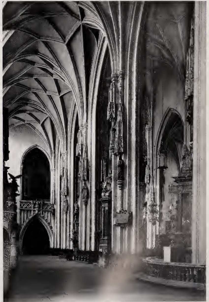
228. Vienna, St Stephen (Cathedral). Interior of the nave, begun 1359
