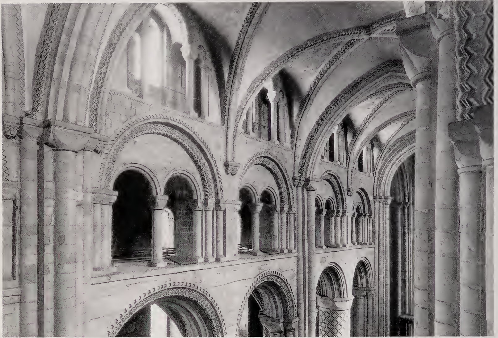
23. Durham Cathedral. Nave c. 1115–33
