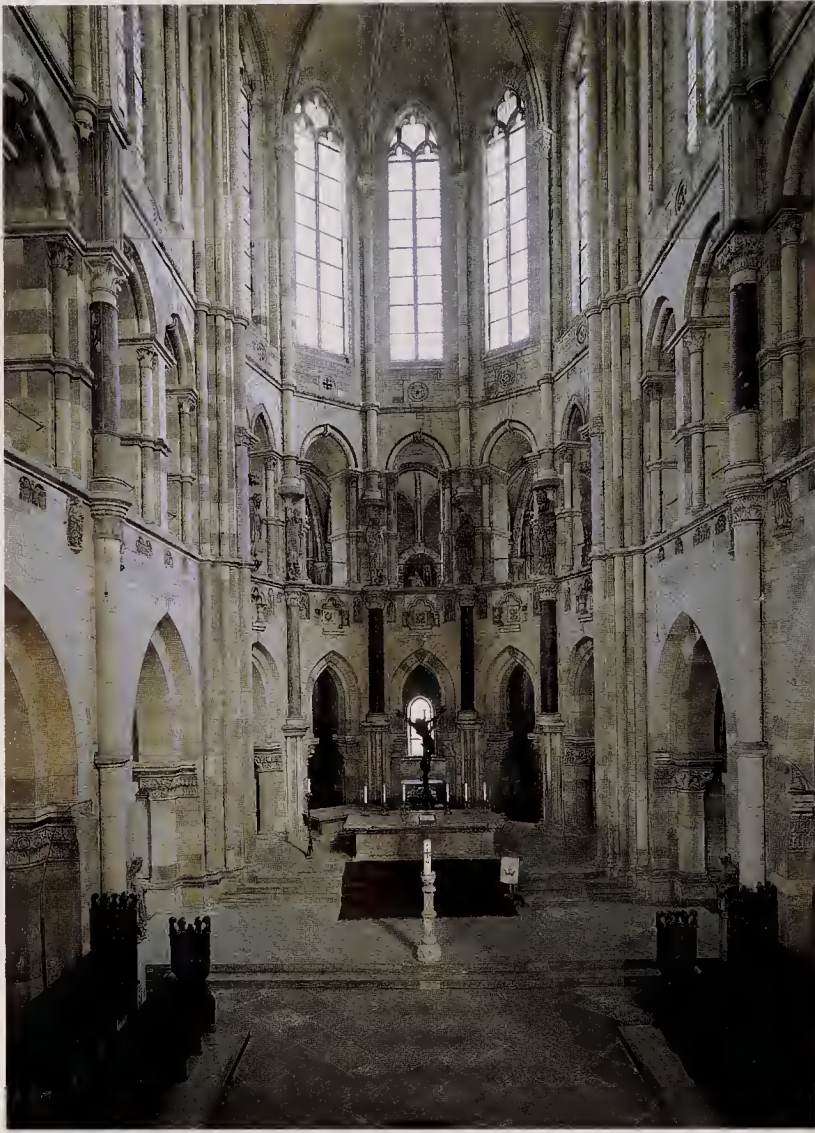
128. Magdeburg Cathedral. Interior of choir, begun 1209
