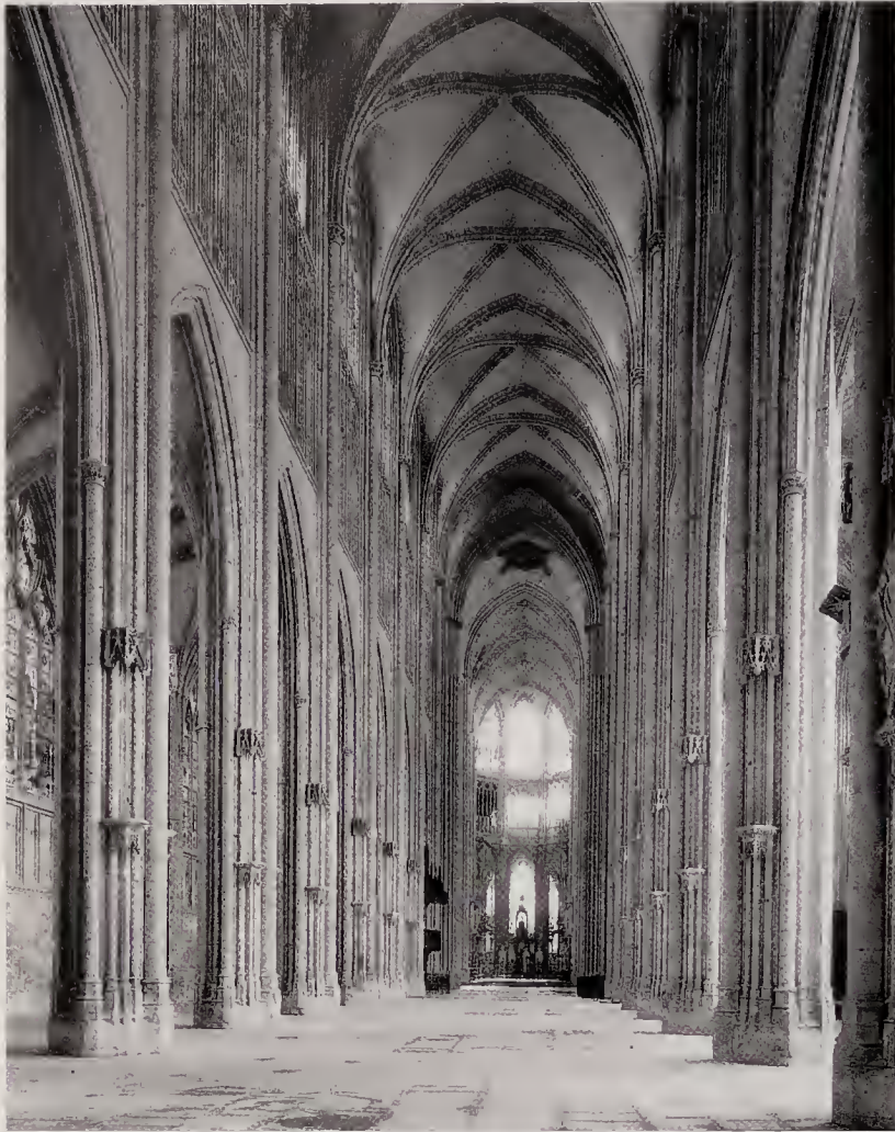
176. Rouen, Saint-Ouen, begun 1318. Interior
