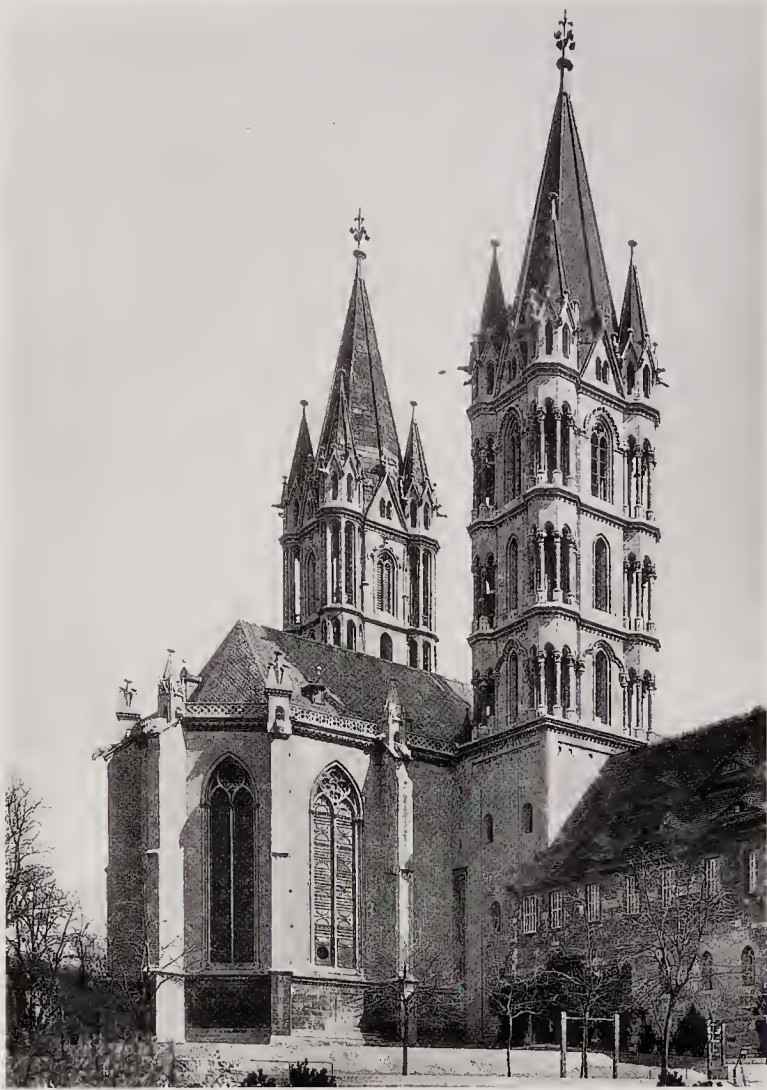
109. Naumburg Cathedral. Exterior of western choir, c. 1250, lower, Romanesque, parts of towers begun c. 1230–40. First Gothic storey of north west tower c. 1250–60
