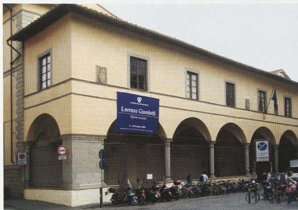
3.14 Ospedale di San Matteo, Florence, begun 1385 under the direction of Romolo del Bandino and Sandro del Vinta, completed 1410.
