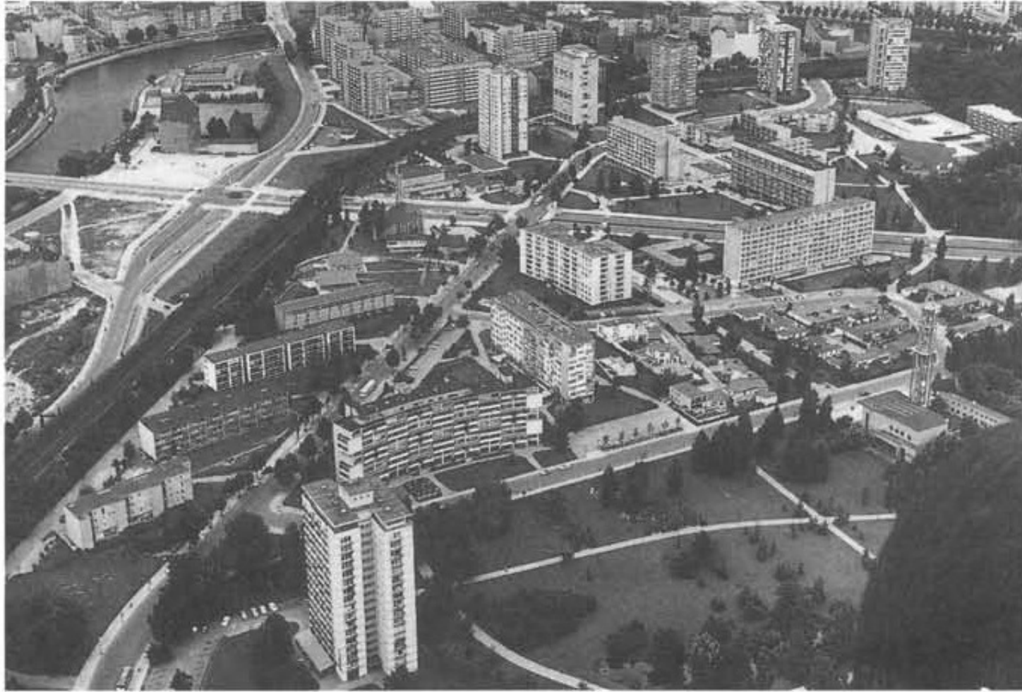
Figure 8.3. Aerial view of the Interbau reconstruction of Berlin's Hansaviertel district in 1962. One edge of the development is bounded by the elevated train tracks, seen as a dark arc extending from the lower left to the upper right side of the photo. The site's other edges abut Berlin's Tiergarten. (Courtesy of Berlin Landesbildstelle, 4 LuA 83 467.)
