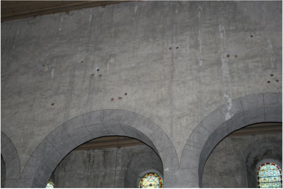
FIGURE 31-1 Saint-Chef-en-Dauphiné, nave wall with acoustic pots. Source: courtesy of the author.
