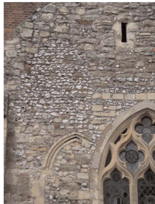
Patching in greensand, limestone, flint and brick make a geological palimpsest of the chapel of the bishop's palace
