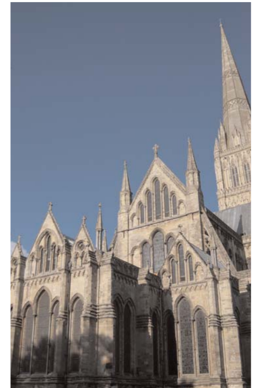
Construction of Salisbury was speeded by the use of many repeated details
