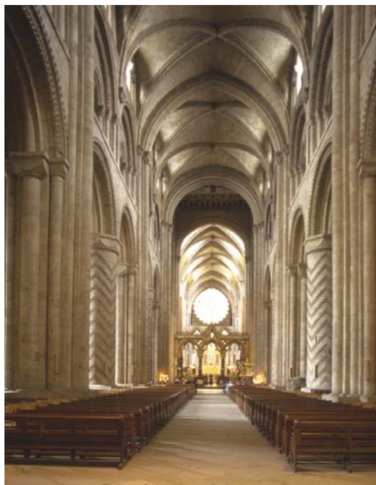
The nave: Durham's rib vaults are among the first in the world
