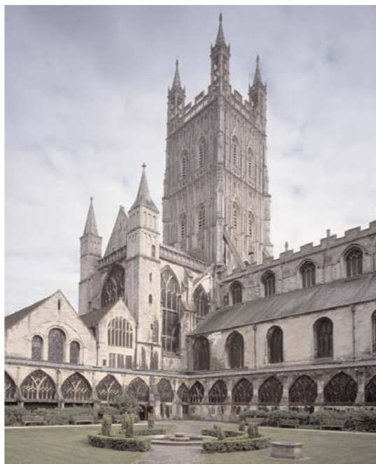
Gloucester's Perpendicular central tower was a magnificent addition to the Norman structure beneath
