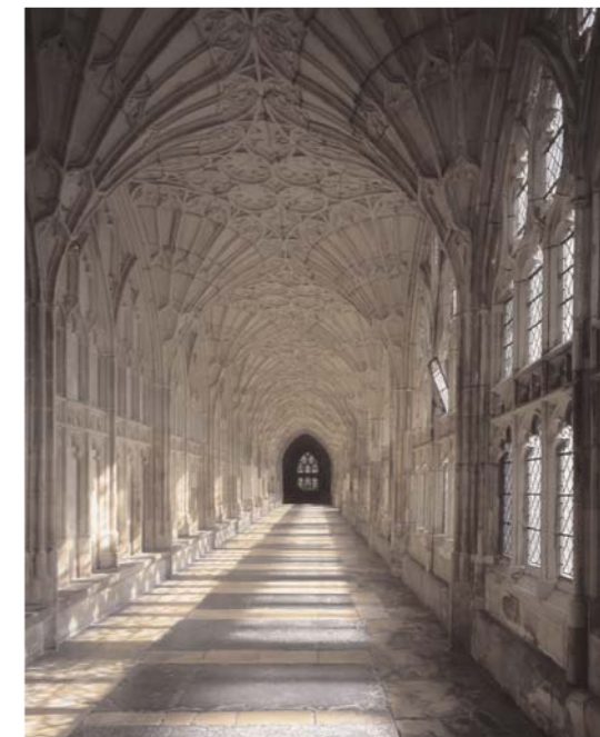
The new technique of fan vaulting was shown off to spectacular effect in Gloucester's cloisters
