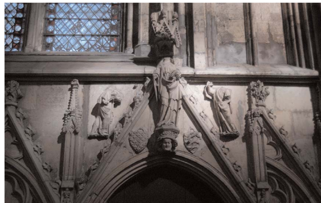
This door in the nave is all that remains of St Sepulchre's chapel, private college of the archbishop
