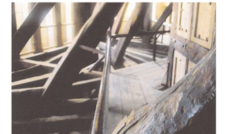
The marks made by labourers' axes are still visible on the timbers supporting Ely Octagon
