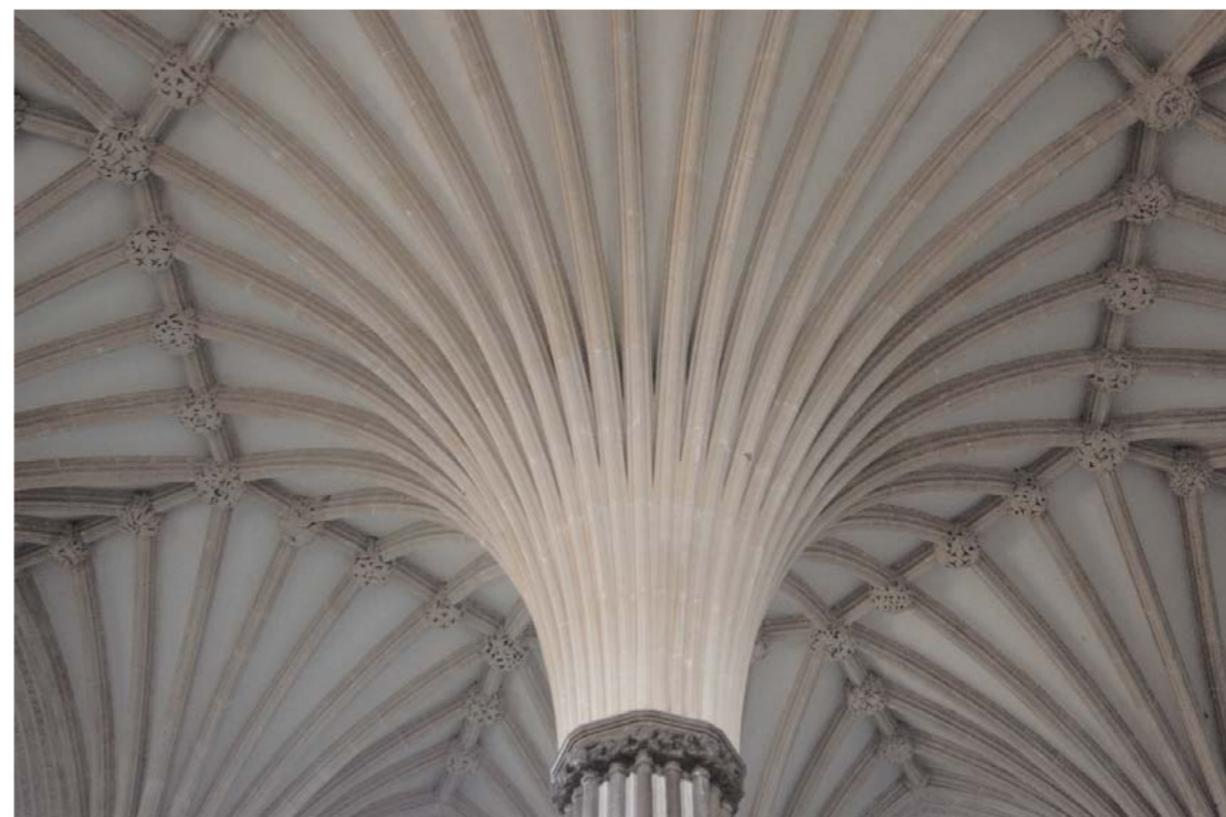
The spectacular tierceron vault of the Wells chapter-house
