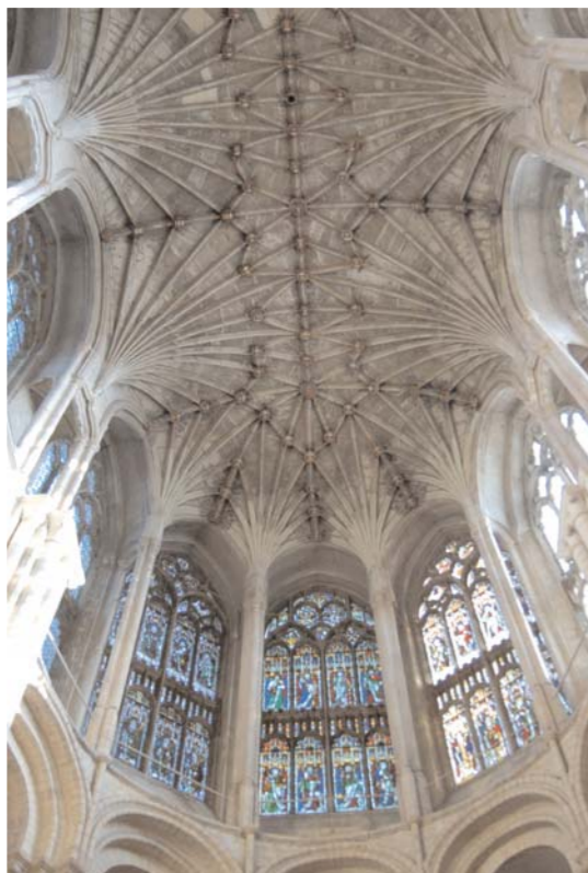
Four hundred years separates the walls and the vault of Norwich's choir
