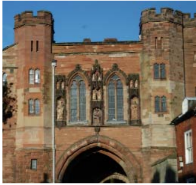
Worcester's Edgar Gate was one of the first of a new breed of heavily-fortified close gatehouse
