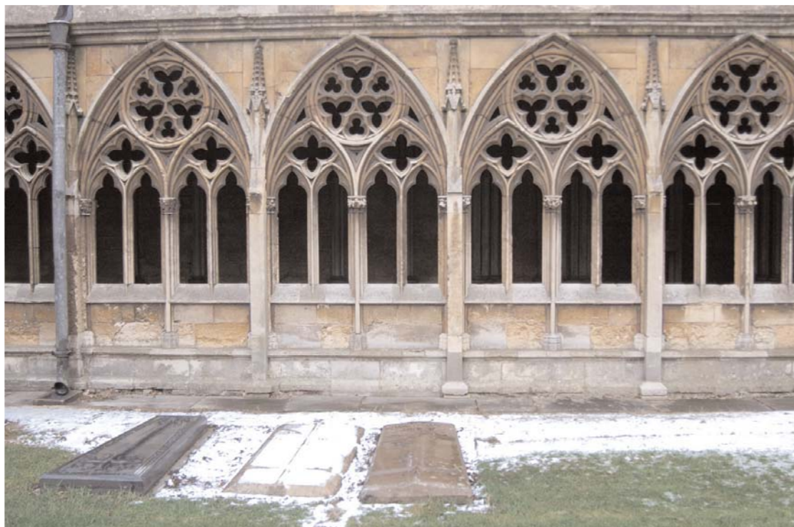
The passage from church to chapter-house and deanery was turned into a cloister from 1296
